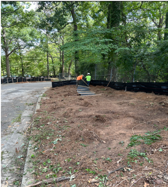
Silt fence install and erosion is near completion
